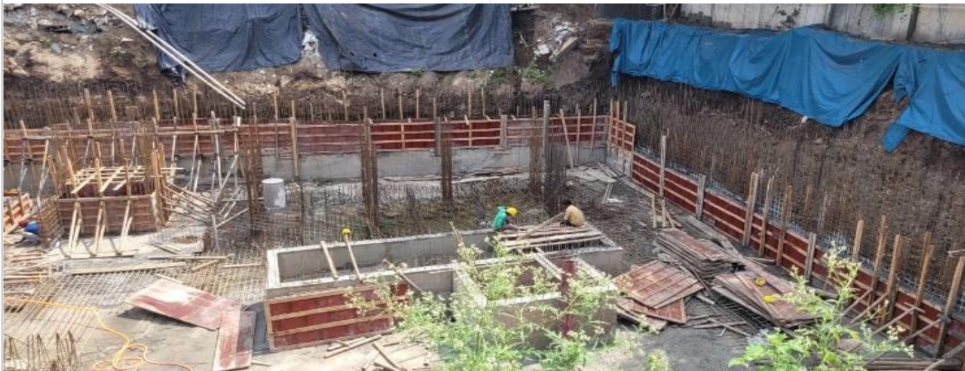
Form work of shear wall
