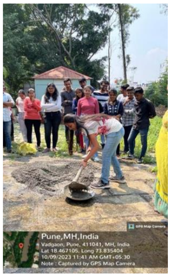
Students learned about proportions for mortar and tried their hand at mortar mixing
