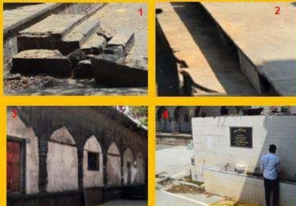
1) Broken stone steps 2) Broken Steps 3) Water Seepage in the wall (Later additions) 4) Water seepage (Water tank is a later addition)
