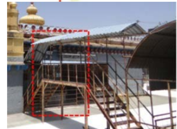
In the new image, the temporary roof shed is attached to the temple. This will be caused of stain, algae and the broken sculptures afterwards.
