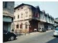
HISTORIC STRUCTURE ON DASTUR MEHER STREET
