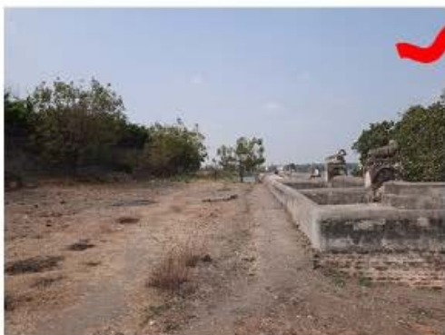
PAVING IN OPEN LAND SPACE , TO AVOID LOSENING OF MORTAR OF RETAINING WALL AROUND BY WATER SEAPAGE
