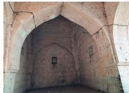
COLOURED STONE LATER ADITION BRICK WALL
