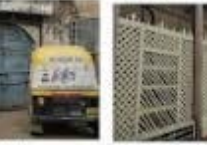
FENCING OF ENTRANCE PORCH
