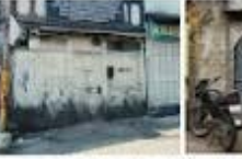
DOORS OF COMMERCIAL SHOP
