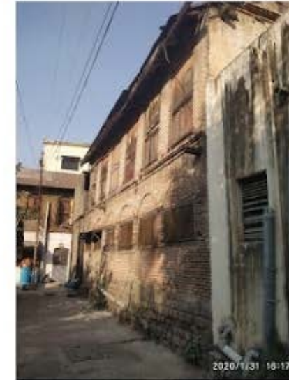
REAR SIDE OF THE STRUCTURE
