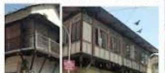
CANTILEVER WOODEN BALCONIES
