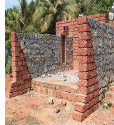
Wall constructed Using Laterite and stone
