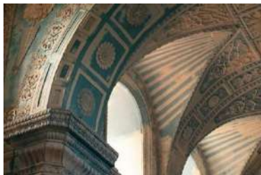
Groin vault (european technology) combined with ornamentation using local motifs in stucco.
