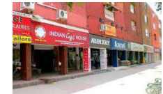
Painting and plastering of façade and columns
