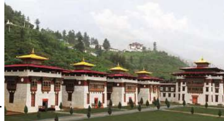
Supreme Court Building, Thimphu
