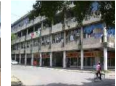
Unauthorized coverage of compulsory veranda
