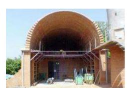
SEMICIRCULAR VAULT, 6 M SPAN BUILT FREE SPANNING IN 6 WEEKS
