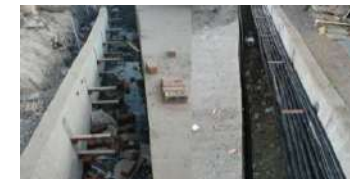
RCC DUCTS FOR UNDERGROUND CABLING
