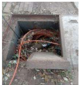
POORLY MAINTAINED TELEPHONE CABLE CHAMBER
