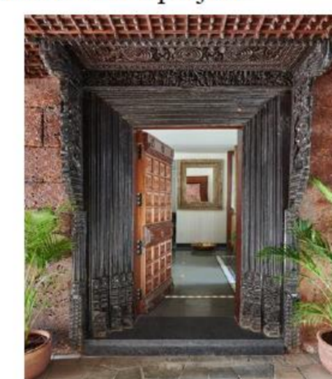
Main entrance door Source : Suleiman Merchant - Maram Bungalow
