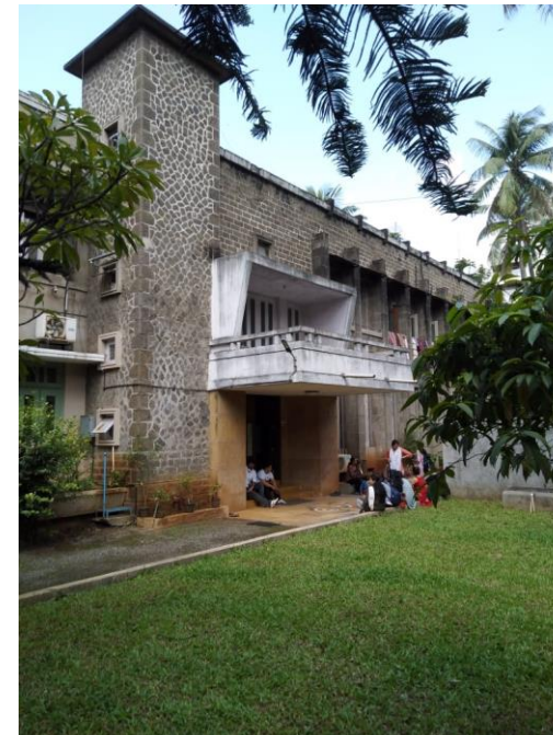
Art Deco style houses on Prabhat Road, Pune.
