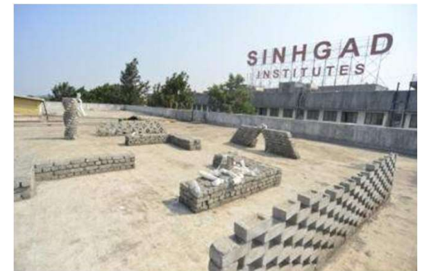
Construction Yard at Terrace
