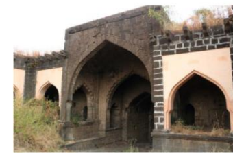
HATHI DARWAZA CEMENT MORTAR JOINTS AND AD-HOC ALTERATION DISTURBING HERITAGE CHARACTER
